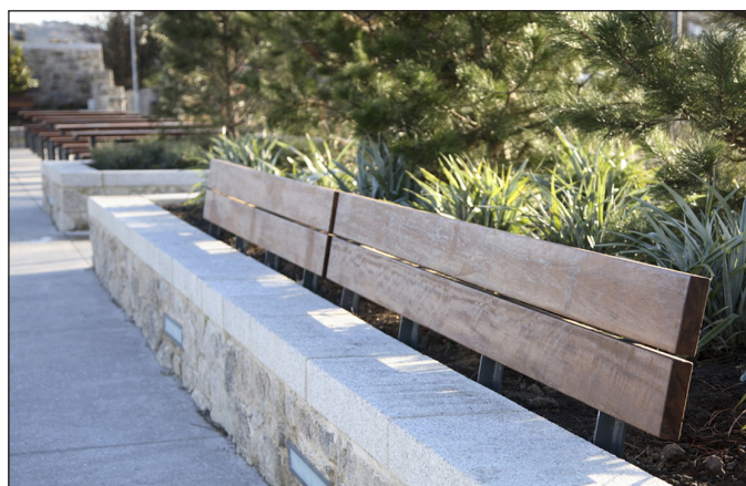
Example of seating walls with masonry top
