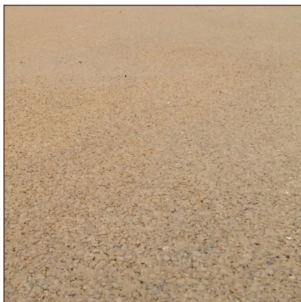
Bitumen macadam surface with coloured wearing course
