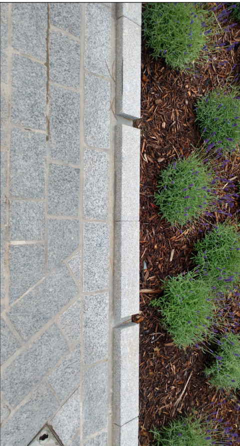
Surface water gully discharging directly into planter bed.
