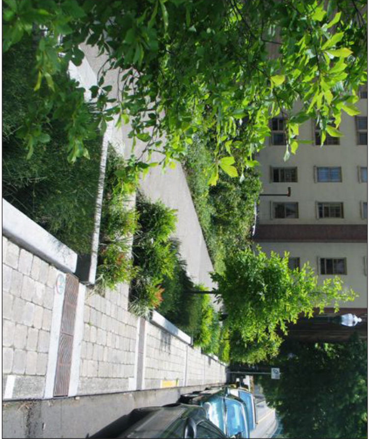
Example of street trees within planting beds incorporating sustainable drainage system
