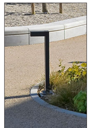
Lighting bollard at edge of planting bed
