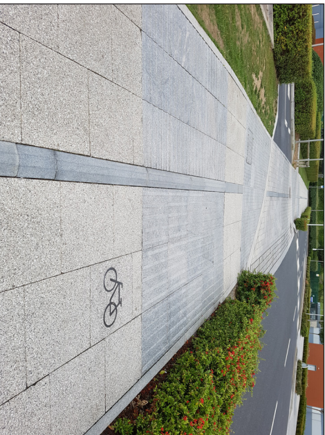
Example of a segregated cycle path integrated with paving and entrance treatments.
