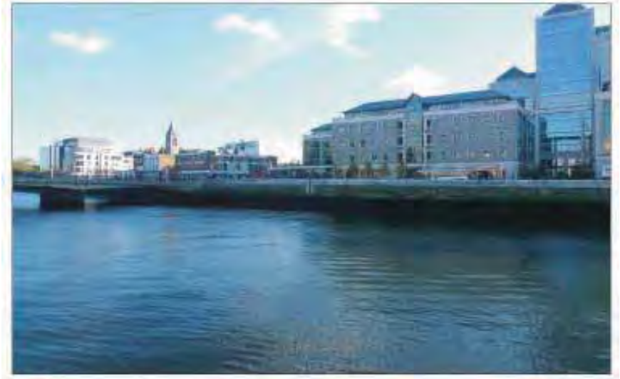
Figure 7 : Proposed view from Custom House Quay. Extract from South Campshire Flood Protection Project, George's Quay, City Quay & Sir John Rogerson's Quay, Dublin 2, EIS, Vol. 3, June 2011
