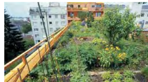
Green Roofs - Sargfabrik, Vienna
