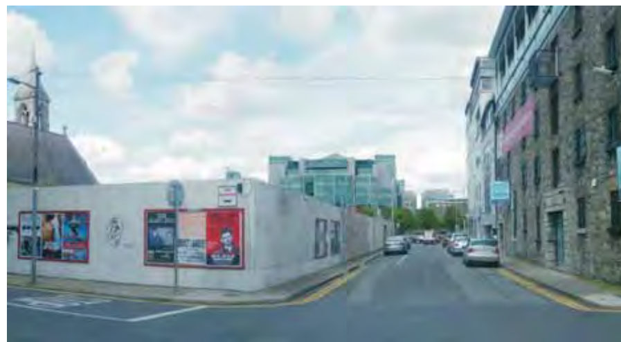
Princes Street South - Existing Situation
