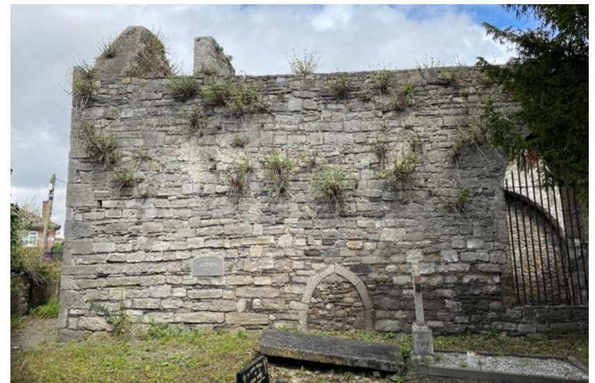
37. View of south wall of side chapel.
