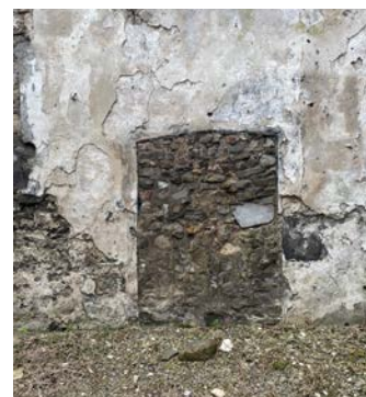
53. Infilled door to side chapel.
