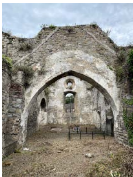
46. West view into nave.
