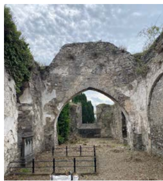
47. East view into chancel.
