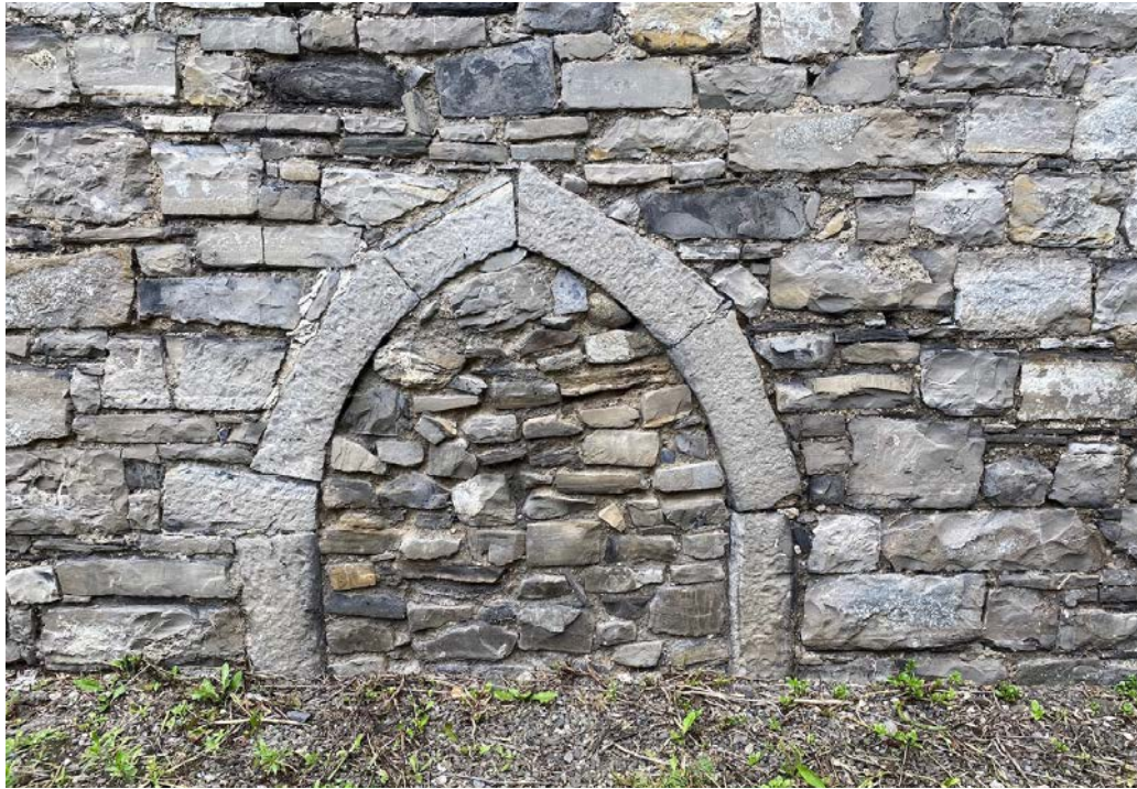
39. Detail of former door into the side chapel facing south in alignment with yew avenue.
