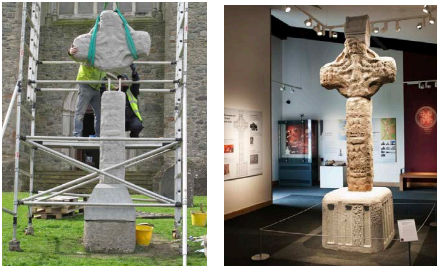
96 & 97. View of replica cross being assembled and Downpatrick high cross relocated into museum and set on new base with new cap.
