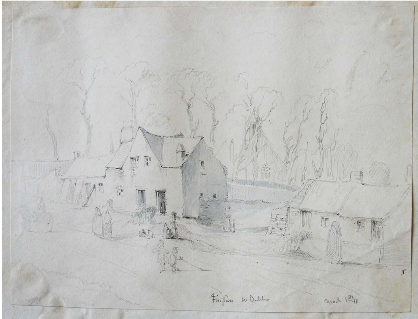
11. Sketch of Barrack Lane by GV Du Noyer in 1841 showing east gable in the background.
