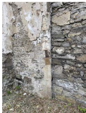
51. Detail of sandstone jambs to side chapel arch.
