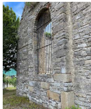
42. West gable window.
