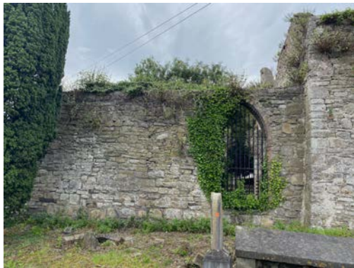
35. North wall of chancel at junction with nave.
