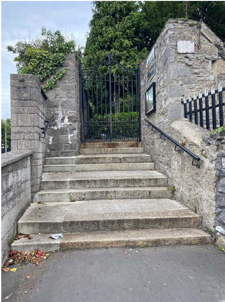
77. View of Barrack Lane (south) gate entrance steps.
