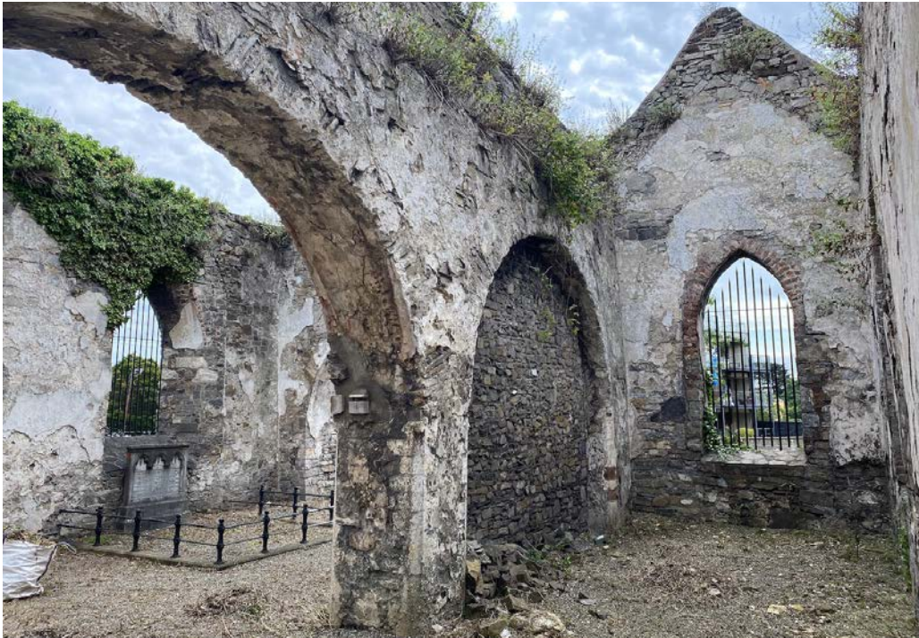
45. View through side chapel arch into nave looking southeast.
