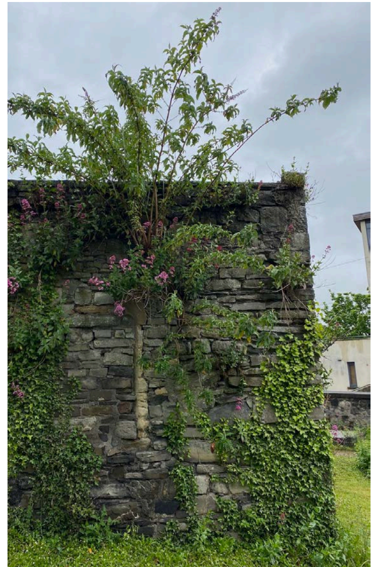
43. View of sandstone window tracery to south end of chancel.
