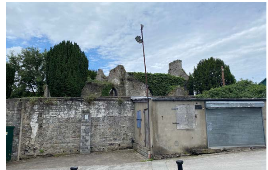
20. View from outside of east wall showing new buttresses.
