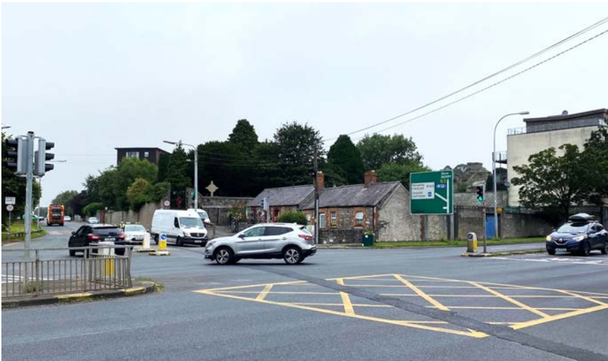
81. View of Nethercross from East Finglas which should be retained.
