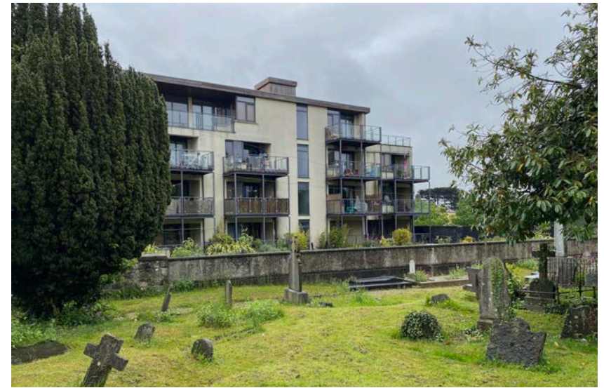
19. View of Fuel Yard Apartments and rebuilt wall section.
