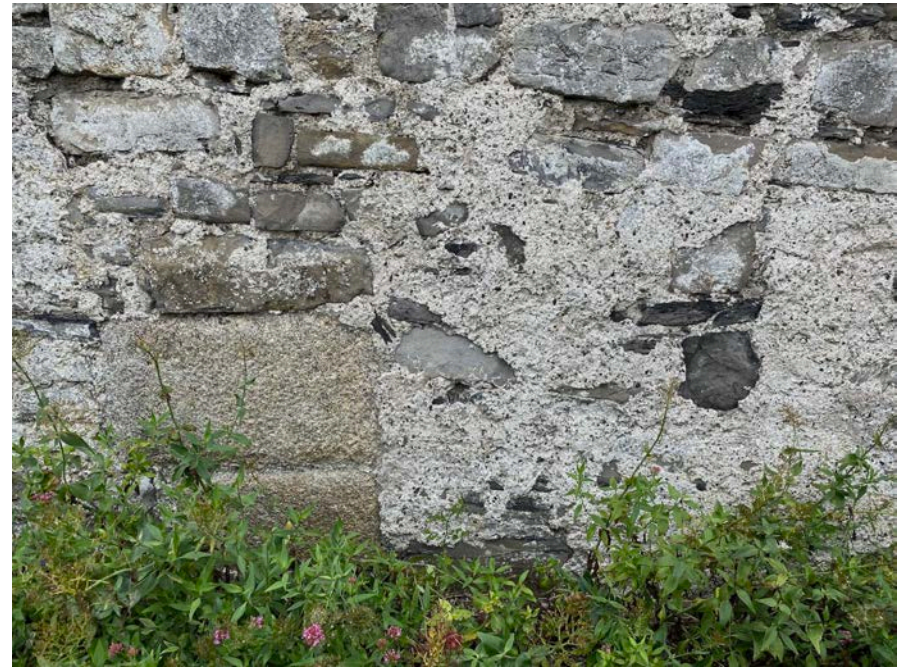
56. Granite ashlar and surviving dash render to west gables.
