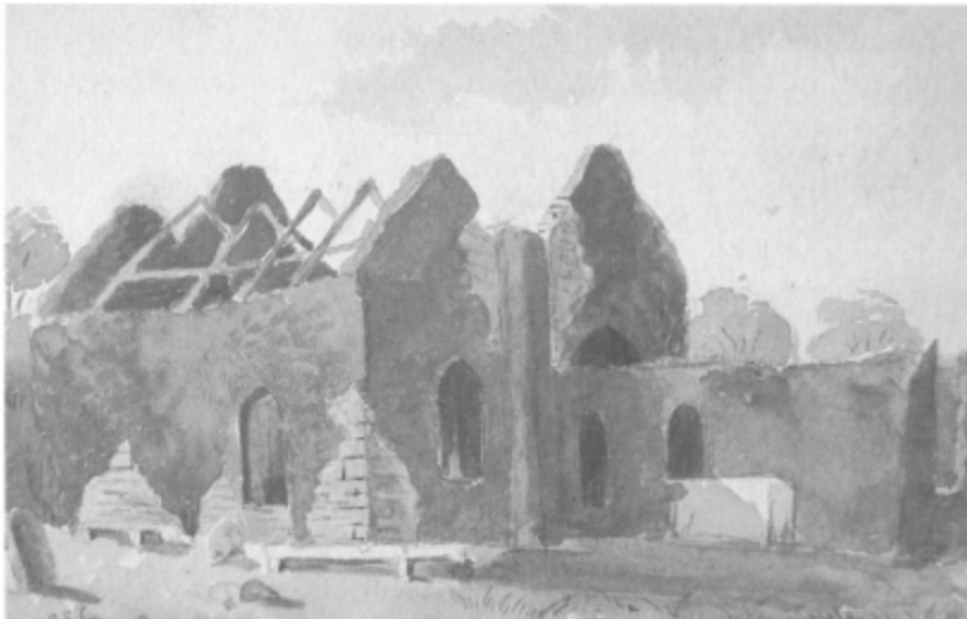
9. Watercolour of church in 1878 By JE Carson showing roof timbers surviving, render shedding and windows missing.
