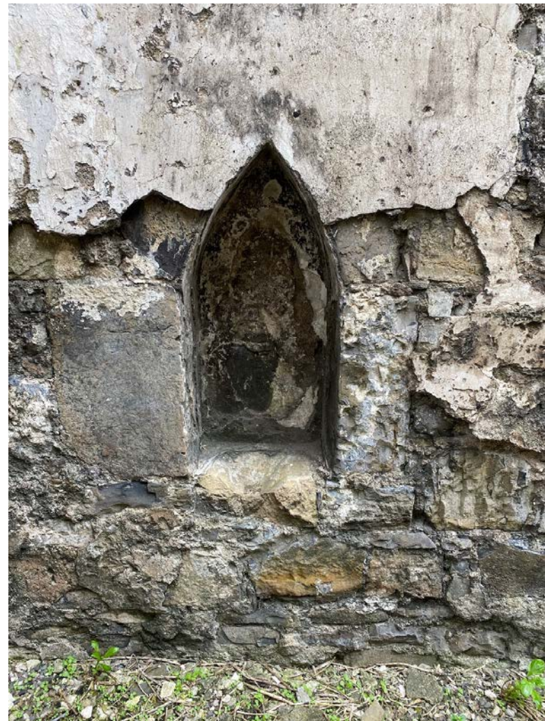
44. Detail of sandstone piscina to side chapel with surviving layers of plaster.
