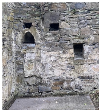
52. Detail of piscina and alcoves to south wall of chancel.
