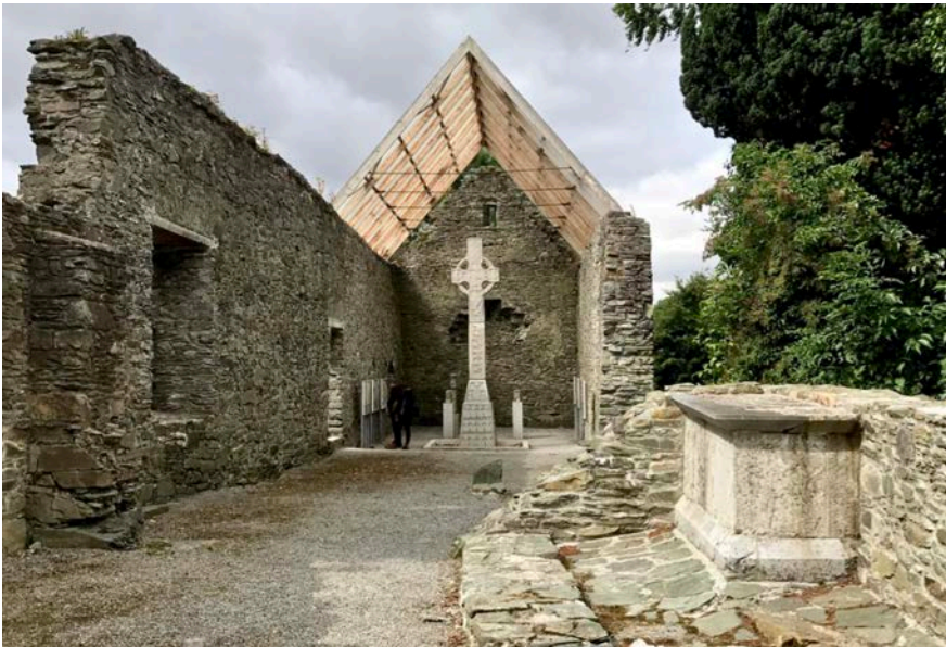
94. View of Moone cross relocated under new timber canopy in ruined church.
