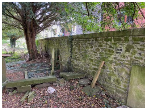
17. View along west boundary wall showing proximity of yew tree.
