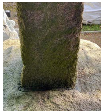
30. Detail of base showing algal growth and granite grains.
