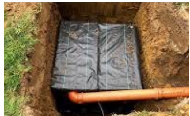
Image: geotextile wrapped plastic crate soakaway being installed
