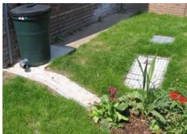
Images: downpipe is directed through water butt and then onwards to the raingarden .
