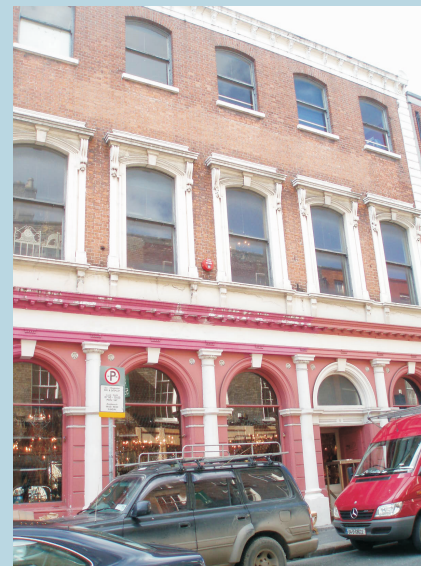
Photo 4.16 No. 114 - 116 Capel Street
