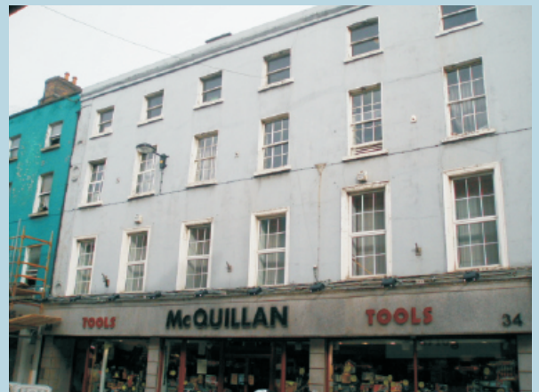
Photo 4.3.1: Mc Quillan's Facade
