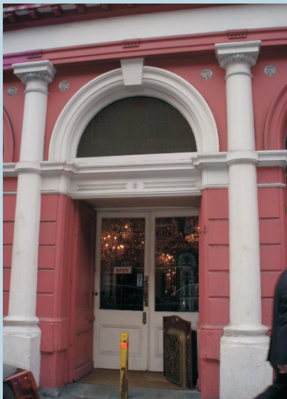
Photo 4.11: Doorcase at Oman Antique Galleries
