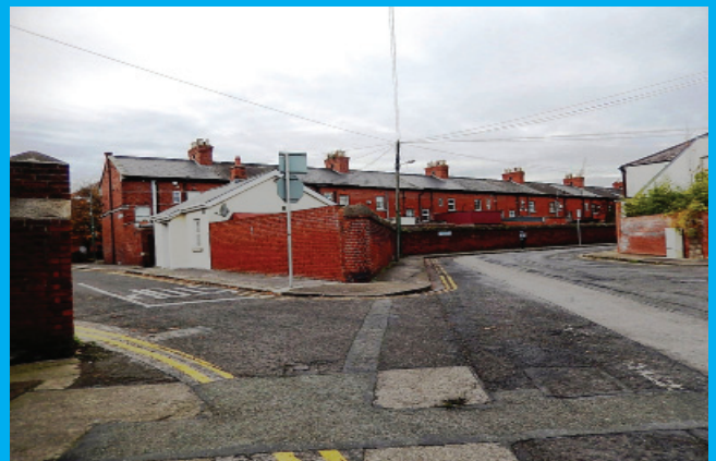
East boundary wall to Avondale Road
