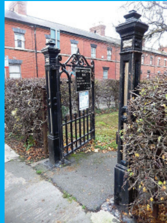
Historic gate to South end
