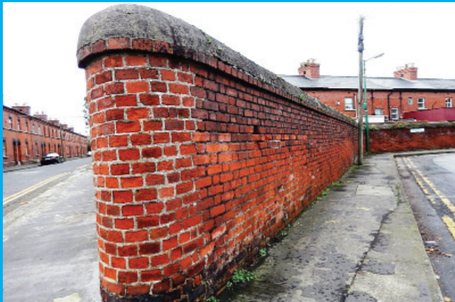
Detail of East boundary wall to Avondale Road
