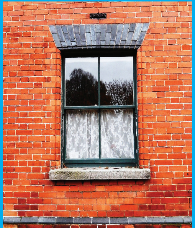
View of historic sash window
