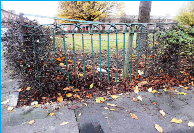
Section of earlier railings to South East corner
