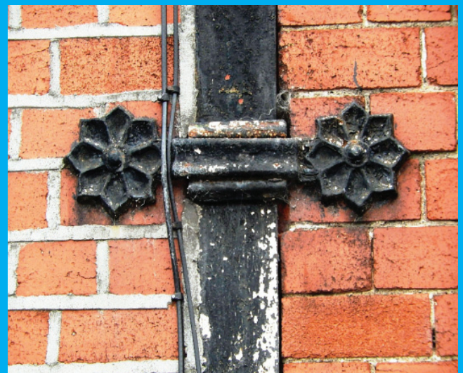
View of recessed cast-iron downpipe detail
