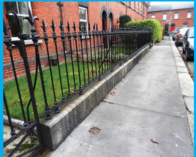
View of railings and gardens to front
