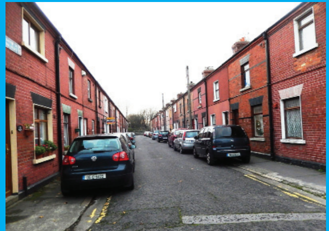
Views east and west of Great Western Villas
