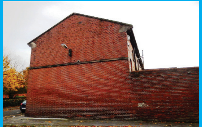
Gable detail of house on west side
