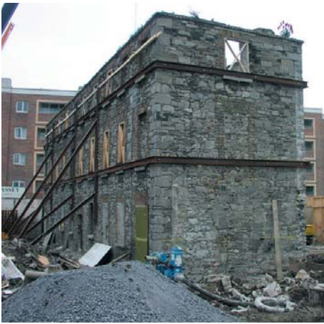
The Widows Alms House during the development of the surrounding site
