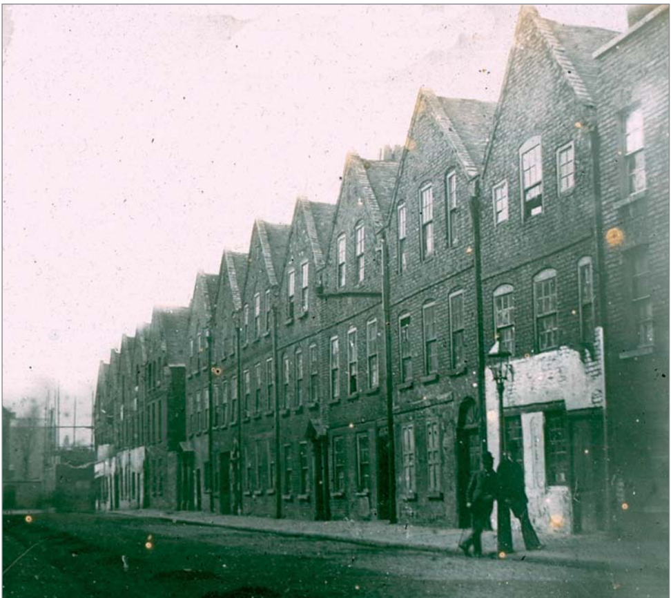
Gable buildings on Chamber St, 1913 (RSAI 'Darkest Dublin')
