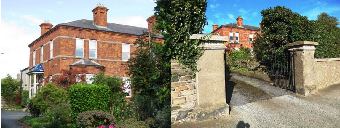
View of 91 Clontarf Road which forms a semi-detached pair with 92 Clontarf Road.
