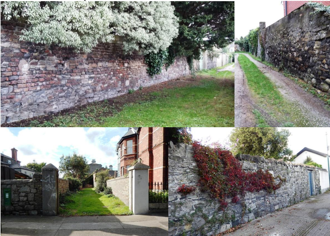
Clockwise from top left, view of section of surviving Clontarf Castle Demesne Wall composed of Brick and Calp Limestone to rear of 31-49 Victoria Road – section of wall shown is the rear boundary of 13 and 15 Kincora Road; view of Calp limestone wall along laneway adjacent to 51 Victoria Road; View of brick and granite wall in laneway between 1 Haddon Road and 92 Clontarf Road; view of surviving section of Calp limestone wall to rear of 37 and 38 Haddon Road.
