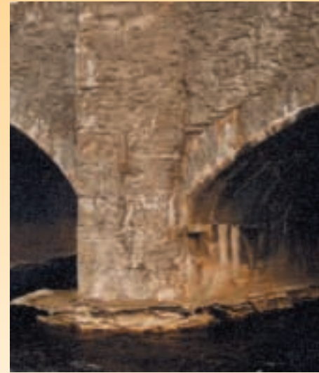
Pressure grouting of bridges can cause encasement and eliminate the crevices used by roosting bats © Bernadette Guest
